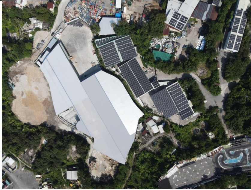
Aerial Photo: Overview of the Site
