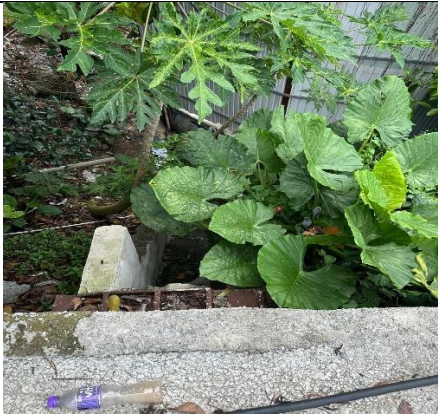
Site Photo 1: Stepped Channel and Existing Stream (5m (W) x5m(H))
