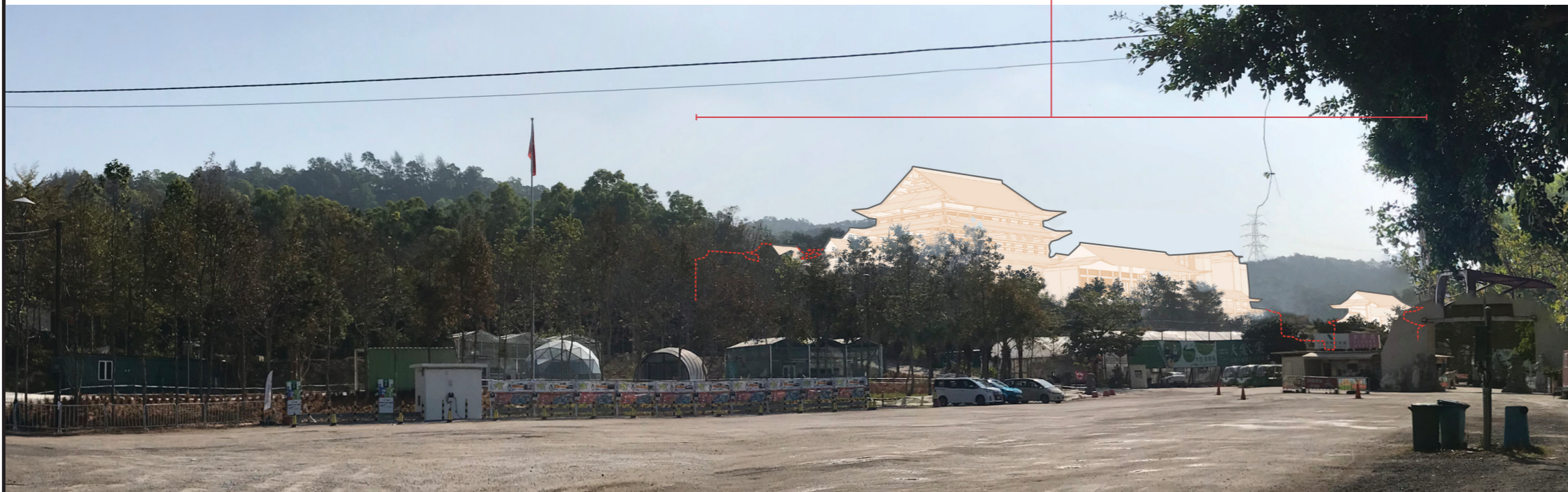
Vantage Point 09: View looking south from visitor car park entrance at Tai Tong Organic Eco Park (Proposed Scheme)
