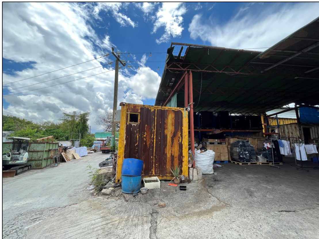
Photo 2.2 Existing Condition of the Site (towards east)
