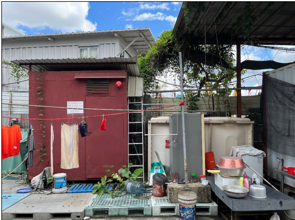
Photo 3.2 Existing FS Pump Room and FS Water Tank within the Site
