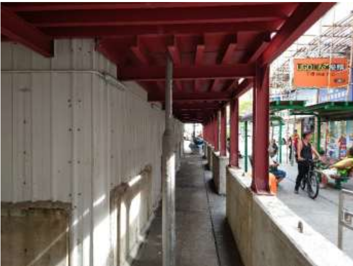
Photo 3: Site perimeter at Fook Hong Street
