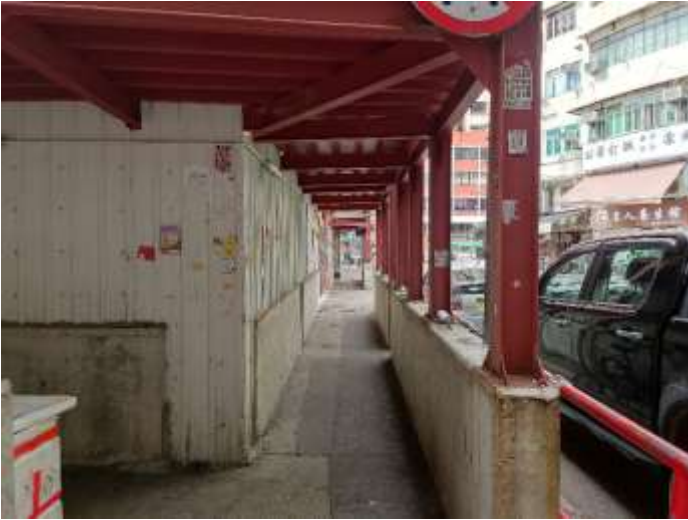
Photo 1: Site perimeter at Yuen Long Pau Cheung Square
