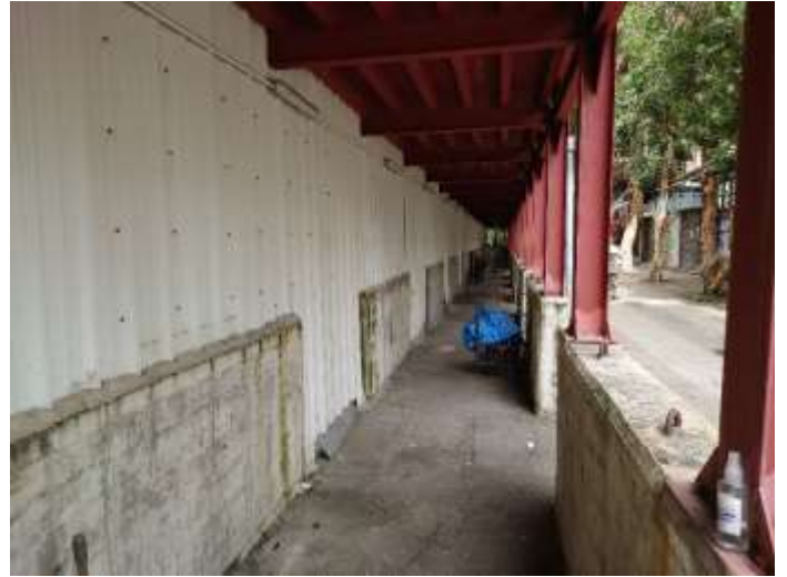
Photo 2: Site perimeter at Fuk Tak Street
