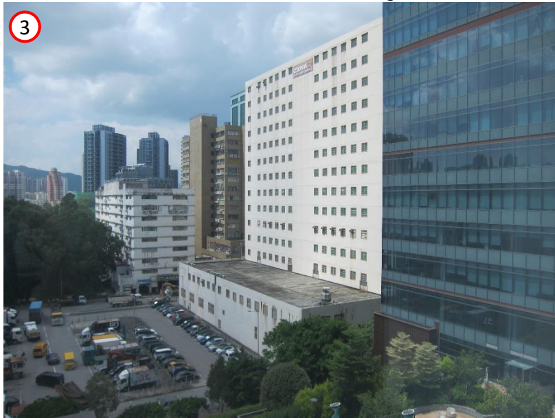
Data Centre and Industrial/I-O Building
