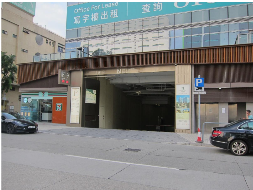
Entrance and exit of car park at G/F
