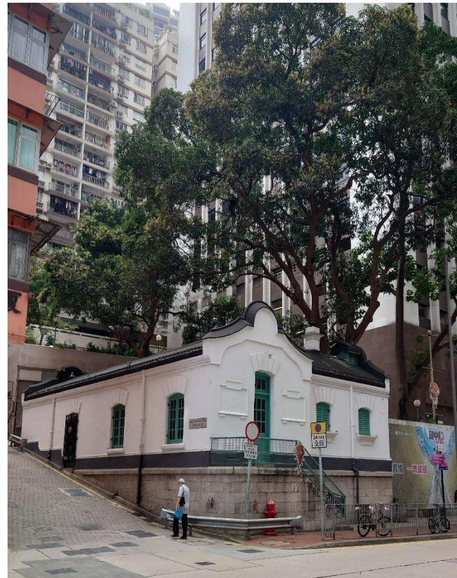
Old Post Office at Wu Chung House [Declared Monument]
