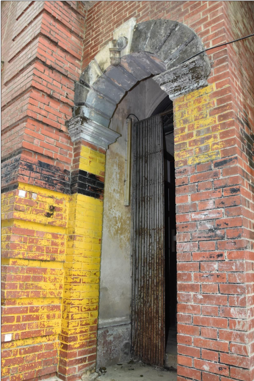
Photo B-03 – Main Building east elevation, the voussoir arch over the side entrance, (21 st March, 2023)
