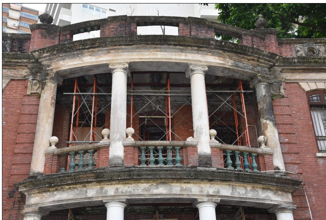
Photo B-10 – Main Building main façade first floor middle part verandah, showing the Ionic columns and the parapet wall in between, (8 th October, 2024)
