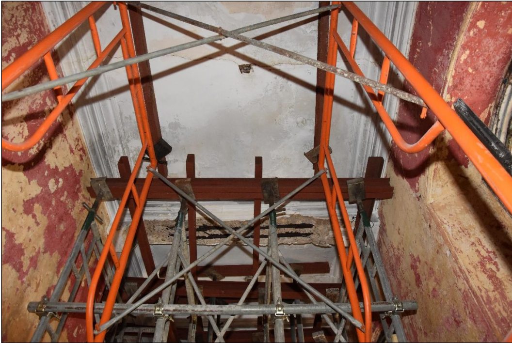
Photo B-51 – Main Building, ground floor, typical stepped ceiling cornice, (8 th October, 2024)
