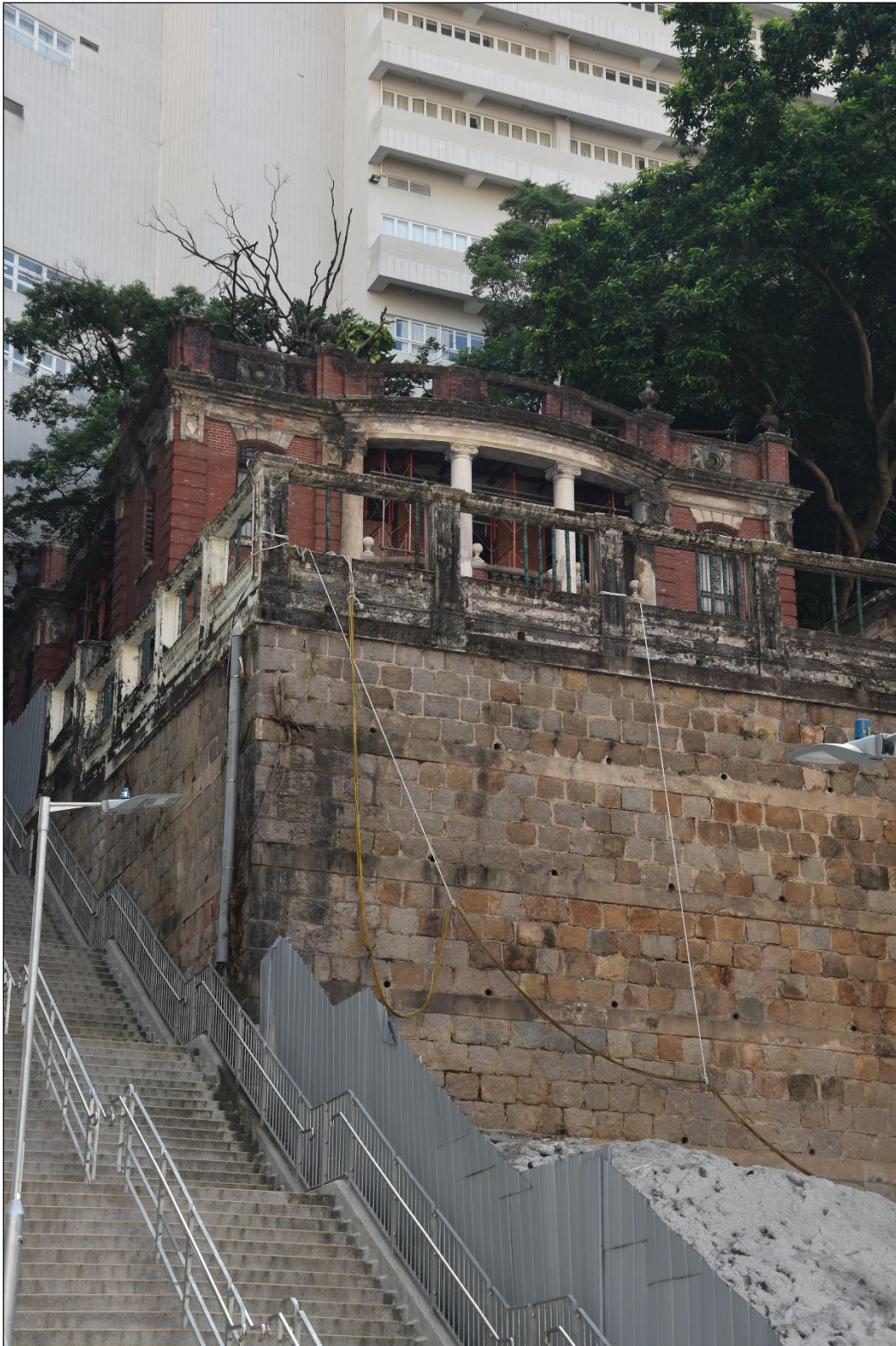
Photo B-08 – The platform formed by granite block retaining wall at the north-west (front) side and south-east (Ship Street) side, (8 th October, 2024)
