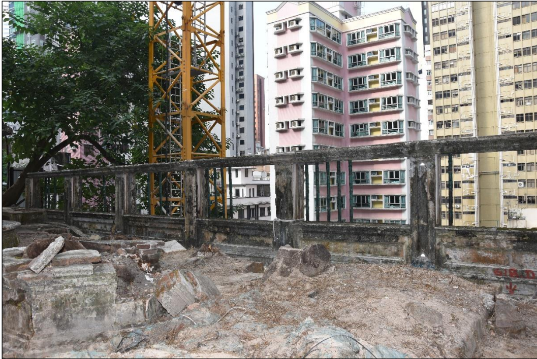
Photo B-61 – The boundary wall above the granite block retaining wall at north-east elevation (facing Queen’s Road East), landscaped garden side, (nearly all the glazed ceramic bamboo shape fencing bars at the upper part have been broken), (8 th October, 2024)
