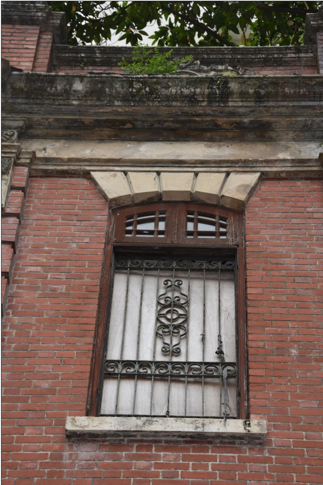
Photo B-06 – Main Building main facade, the window on first floor east side with the wrought iron window grille, (21 st March, 2023)
