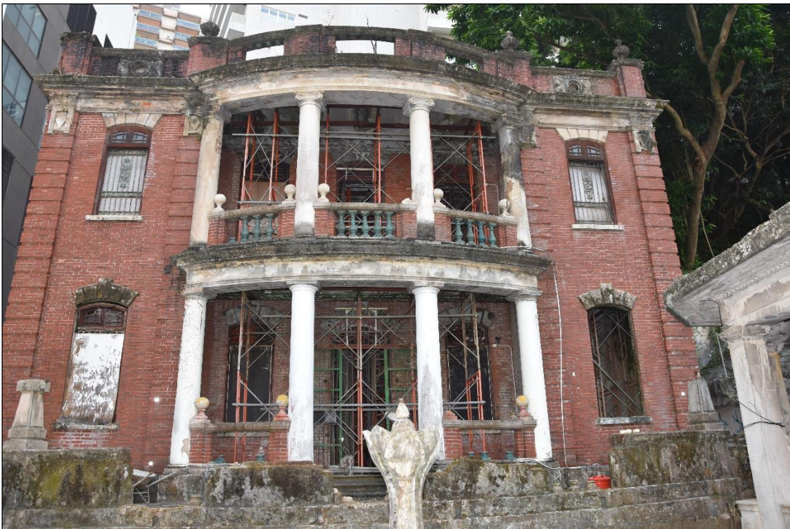
Photo A-02 – Nam Koo Terrace, Main Building main facade, (8 th October, 2024)
