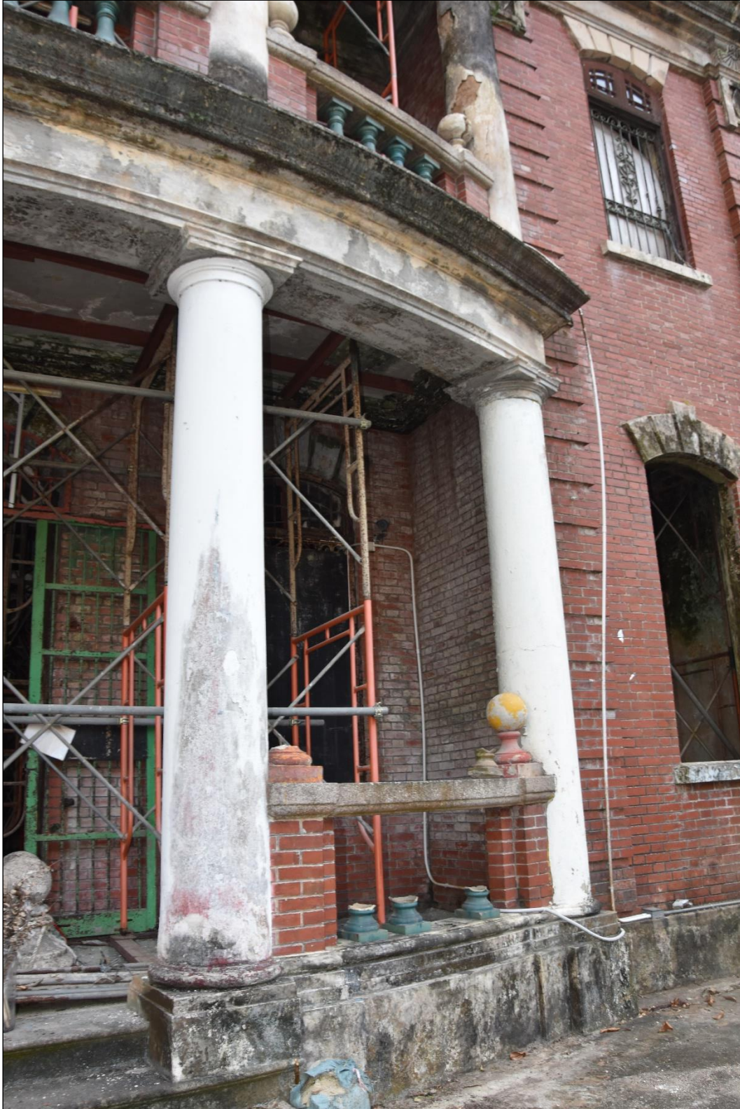
Photo B-12 – Main Building main façade ground floor west part of recess entrance porch, showing the Doric Ionic columns and the parapet wall in between, (the 4 nos. glazed ceramic bottle shape balusters are all broken), (8 th October, 2024)
