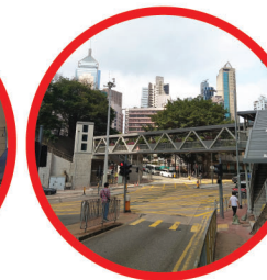
4. Junction Improvement Works at Kennedy Road / Queen's Road East (Construction of footbridge included)
