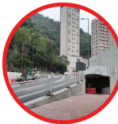
5. Road widening and continuous pavement on both sides of Kennedy Road
