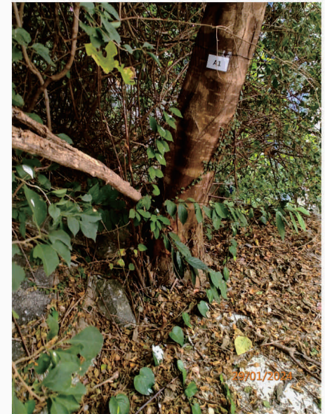
A1 - Tree at the Edge of Retaining Wall (F)
