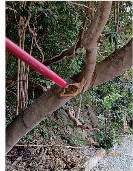
T66 - Heartwood Damage in Trunk (F)
