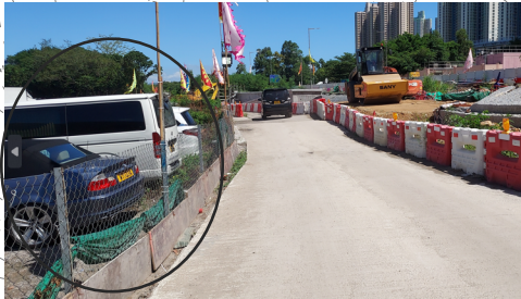
Photo 03 existing car parking area is fenced off from adjacent access road
