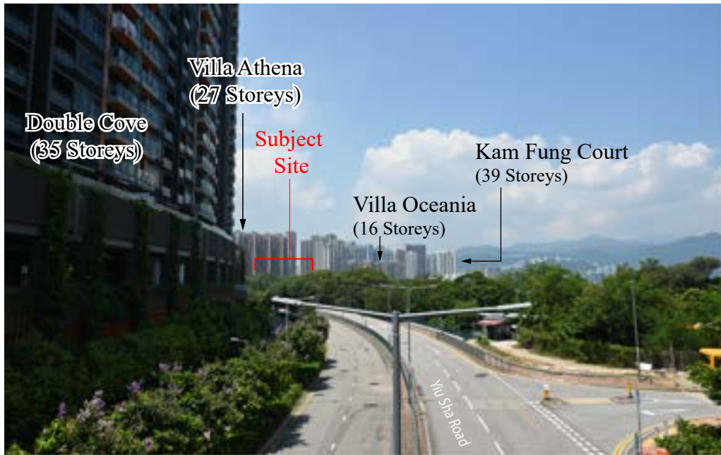
Photo 2A Existing View
