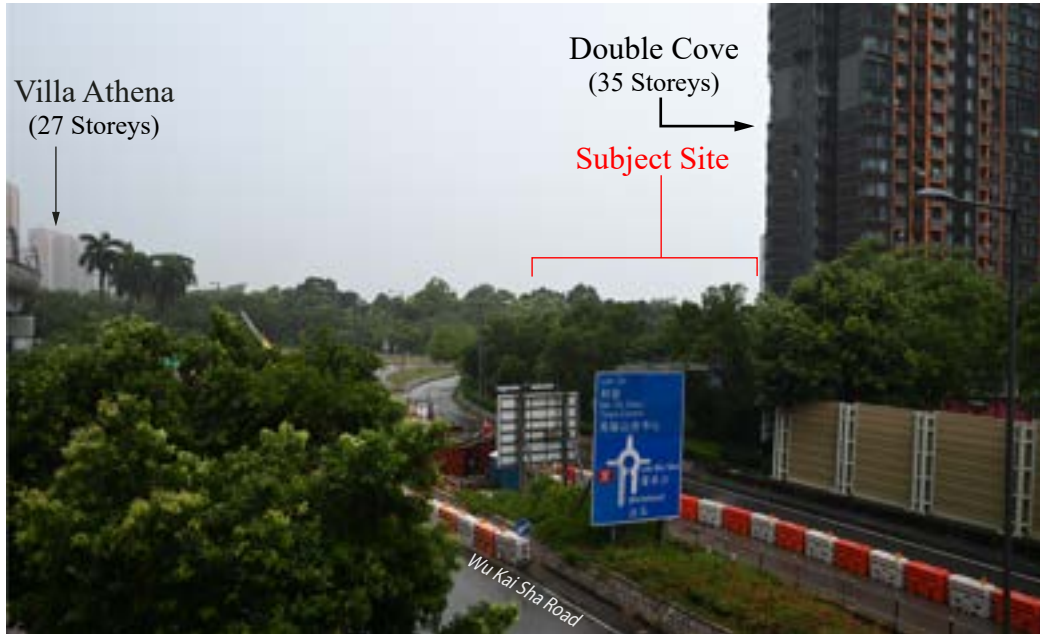
Photo 1A Existing View
