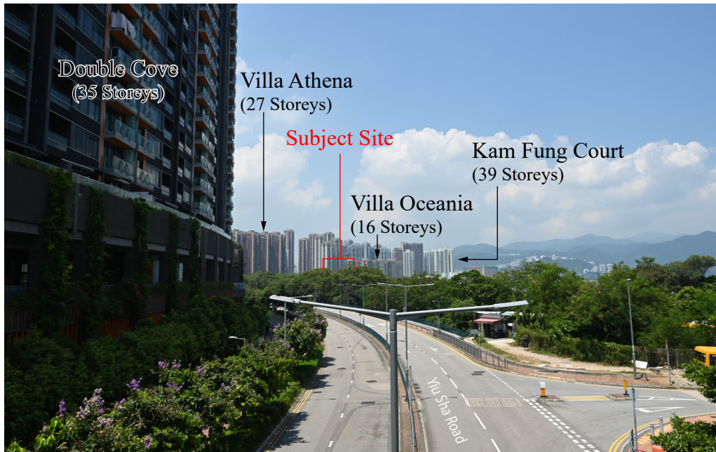
Photo 2A Existing View
