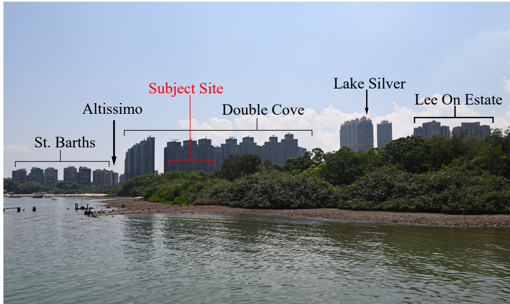
Photo 5A Existing View
