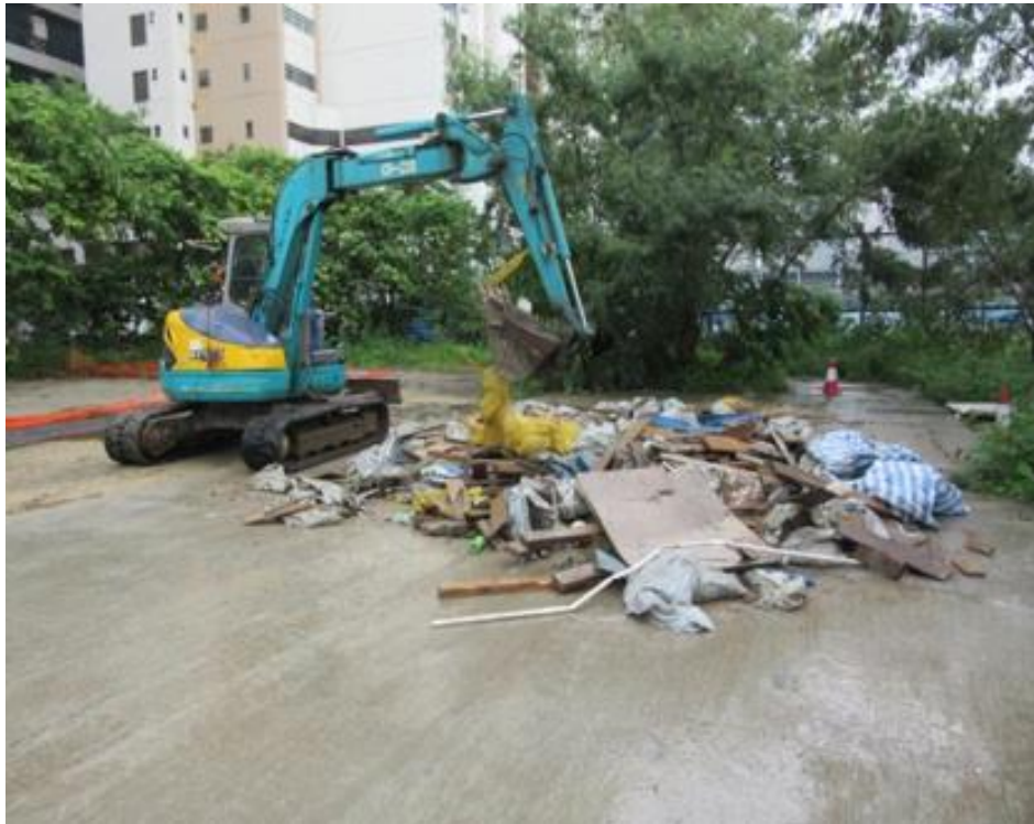
Photo 4 Using backhoe to even the debris
