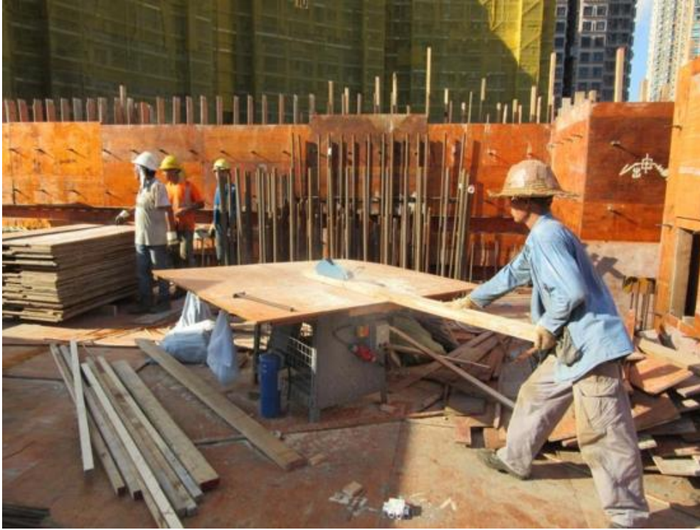
Photo 2 Site visit at Site B
