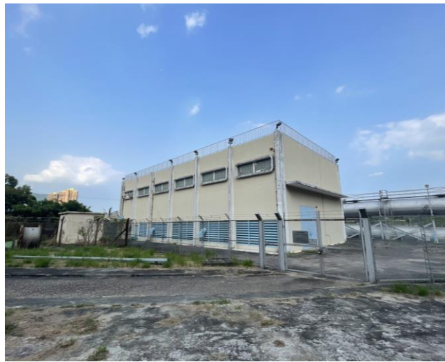
① River Ganges Pumping Station
