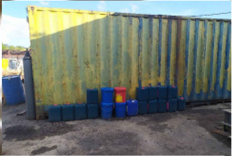
Waste oil container found (improper storage)
