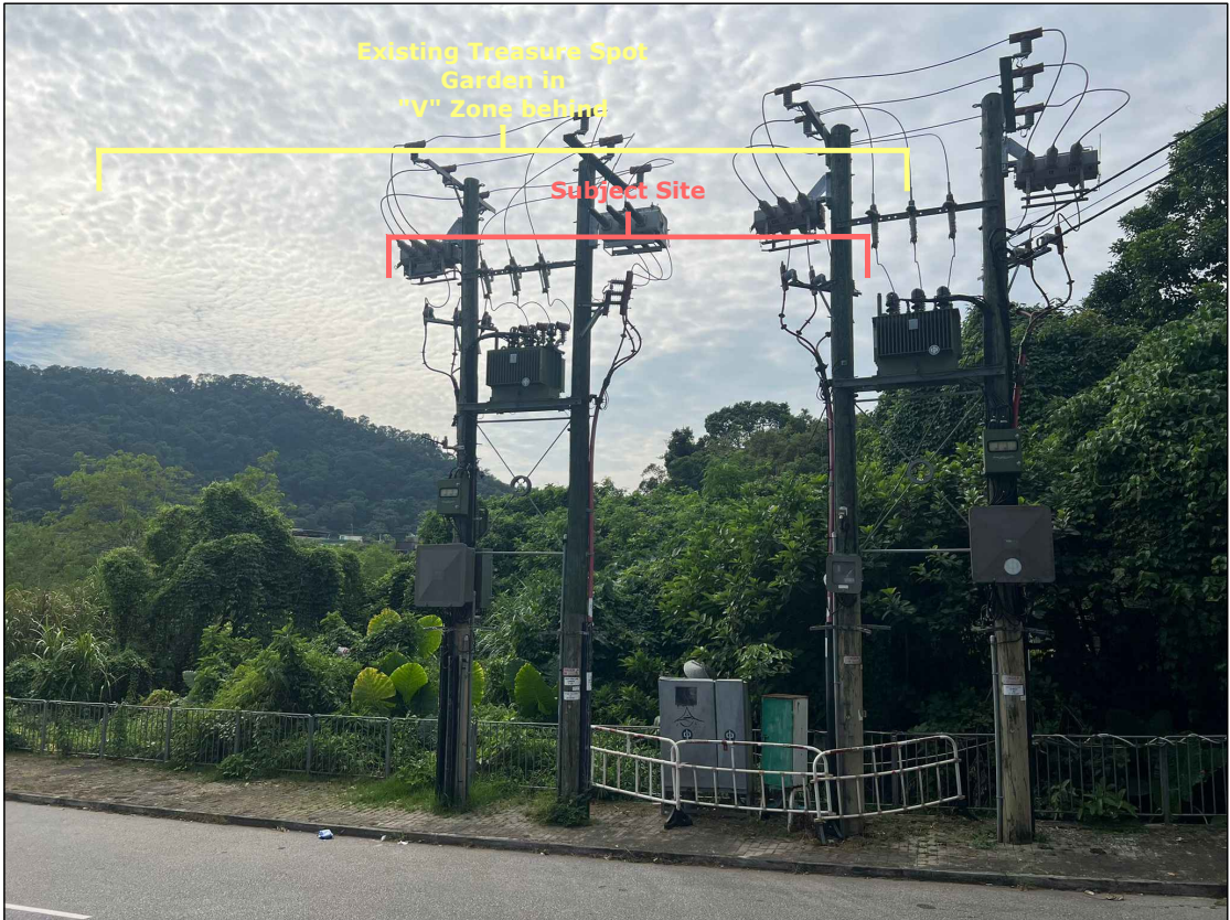
Existing condition (Scheme A)
