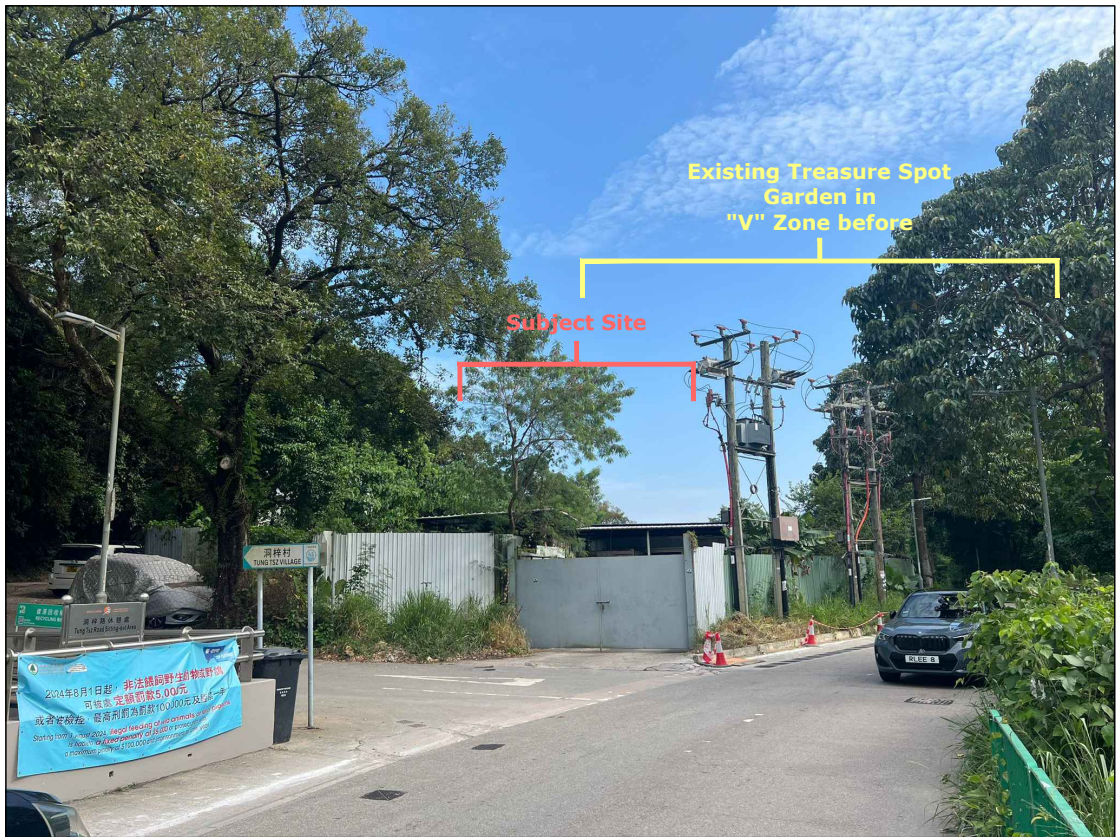
Existing condition (Scheme A)
