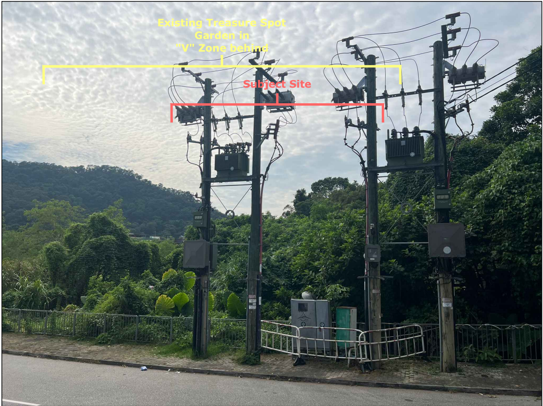
Existing condition (Scheme A)
