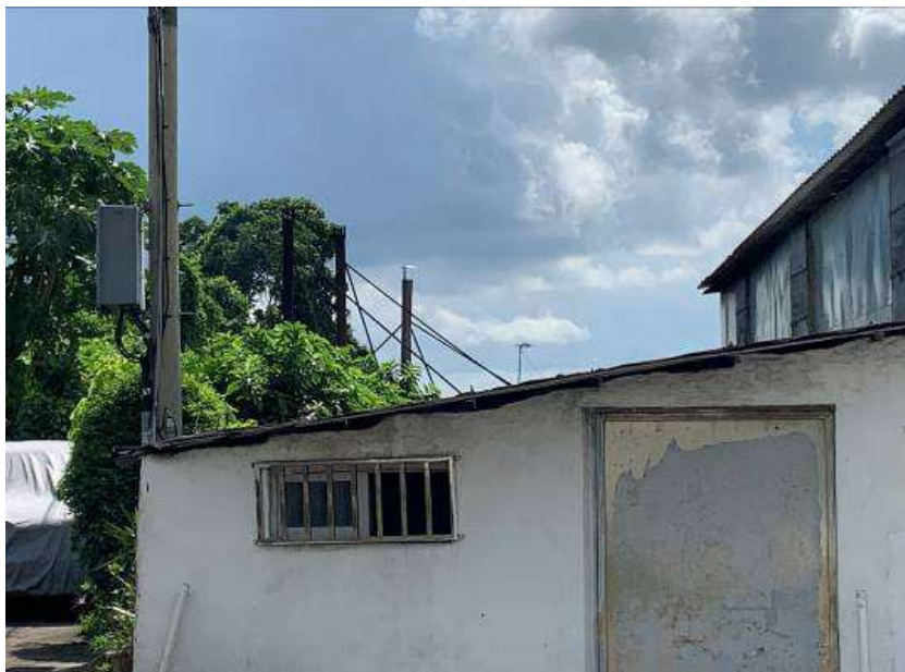
Photo of the 3 chimneys at Koon Yick taken at 10:00am on July 6 th 2023
