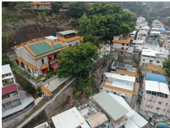
Photo 9: Major level difference and mature trees.
