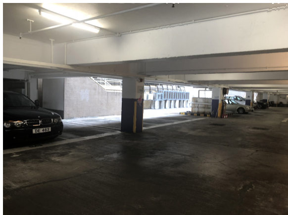
Photo 15: Carpark at Tai Wo Plaza
