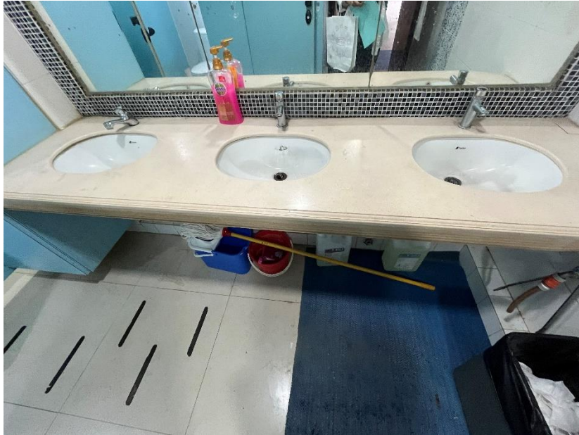
Women's Toilet with washing basins (3 nos.) and water closets (4 nos.)
