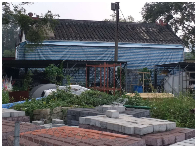
Photo 14: Regular restoration and preservation works.
