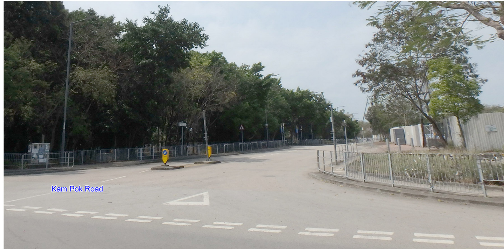
VIEWPOINT VP3 FROM JUNCTION OF KAM POK ROAD / CASTLE PEAK ROAD - EXISTING SITUATION
