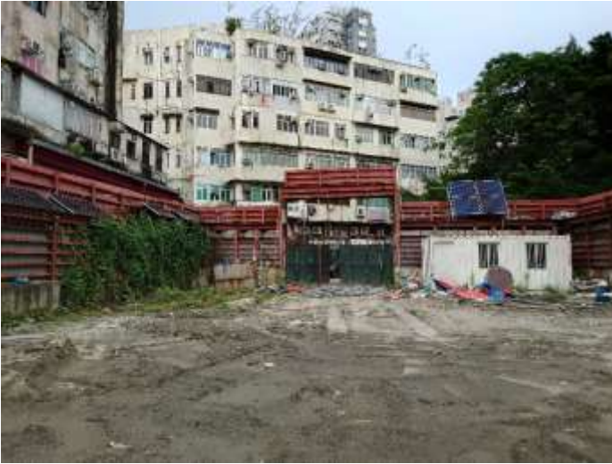
Photo 7: General view of the site
