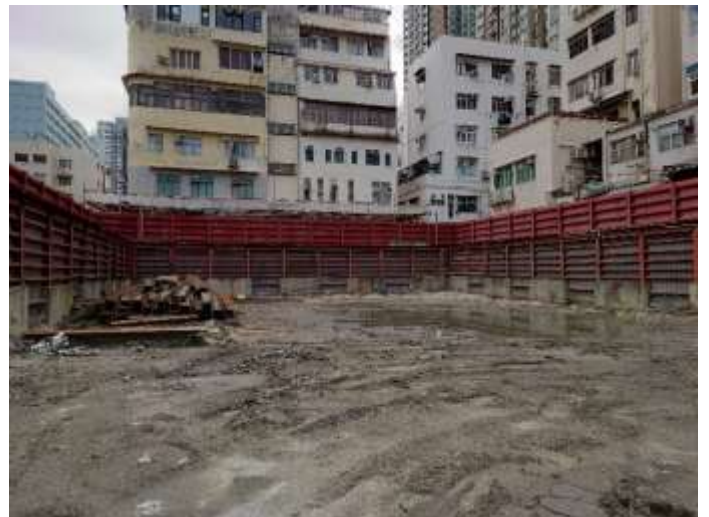
Photo 12: No oil stain is observed on the ground
