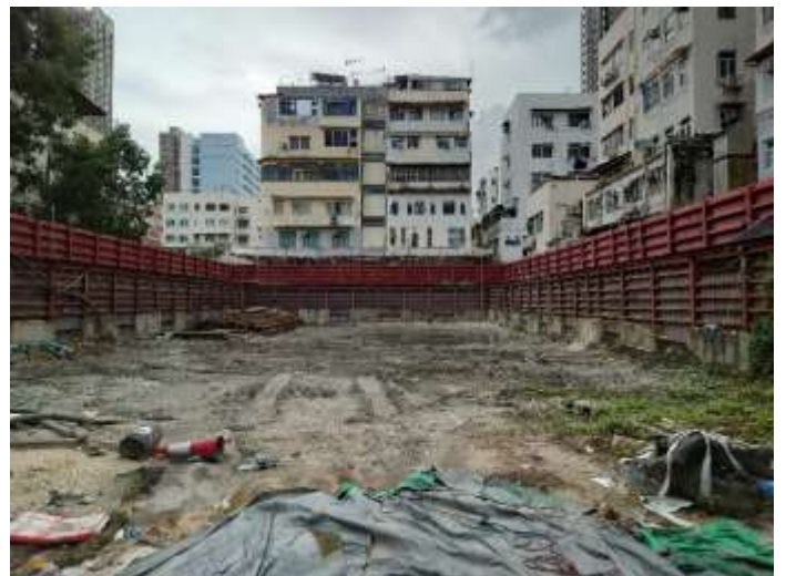
Photo 6: general view of the site
