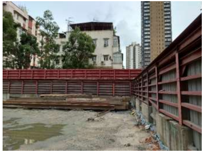
Photo 10: Temporary storage of H beam at the southwest of the site
