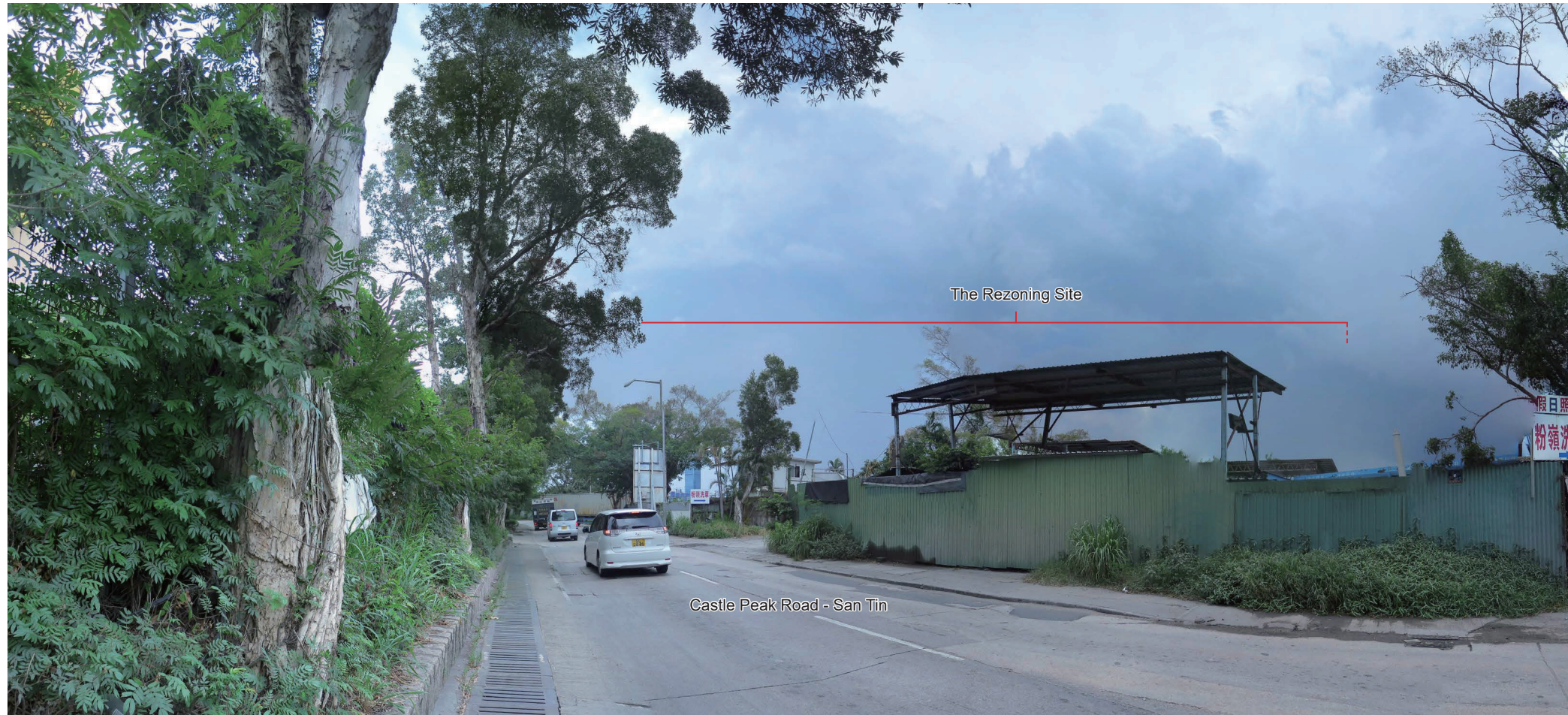
Existing View View north-west from Castle Peak Road - San Tin
