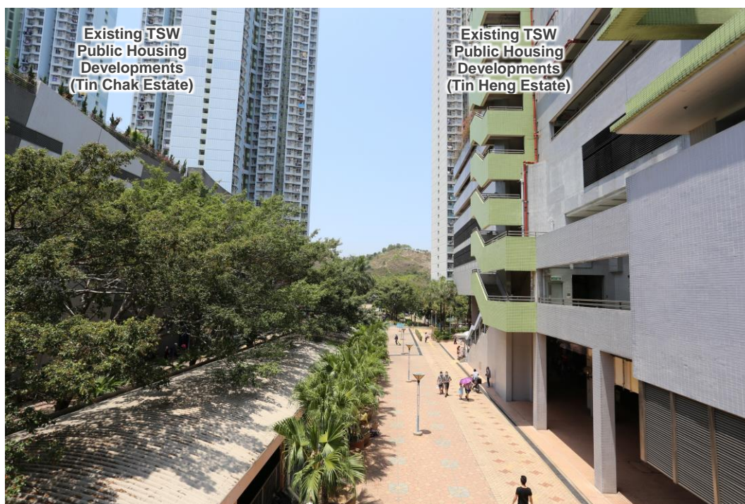
Existing View from the Footbridge at the Open Space Spine within TSW Public Housing Estates
