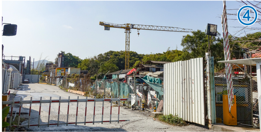
The Application Site (to the right of the access road)
