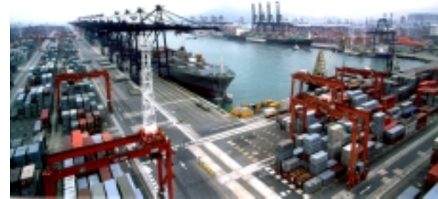
• 葵涌港口設施。 Port facilities at Kwai Chung
