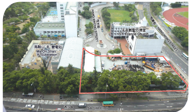
恆光街 Hang Kwong Street
