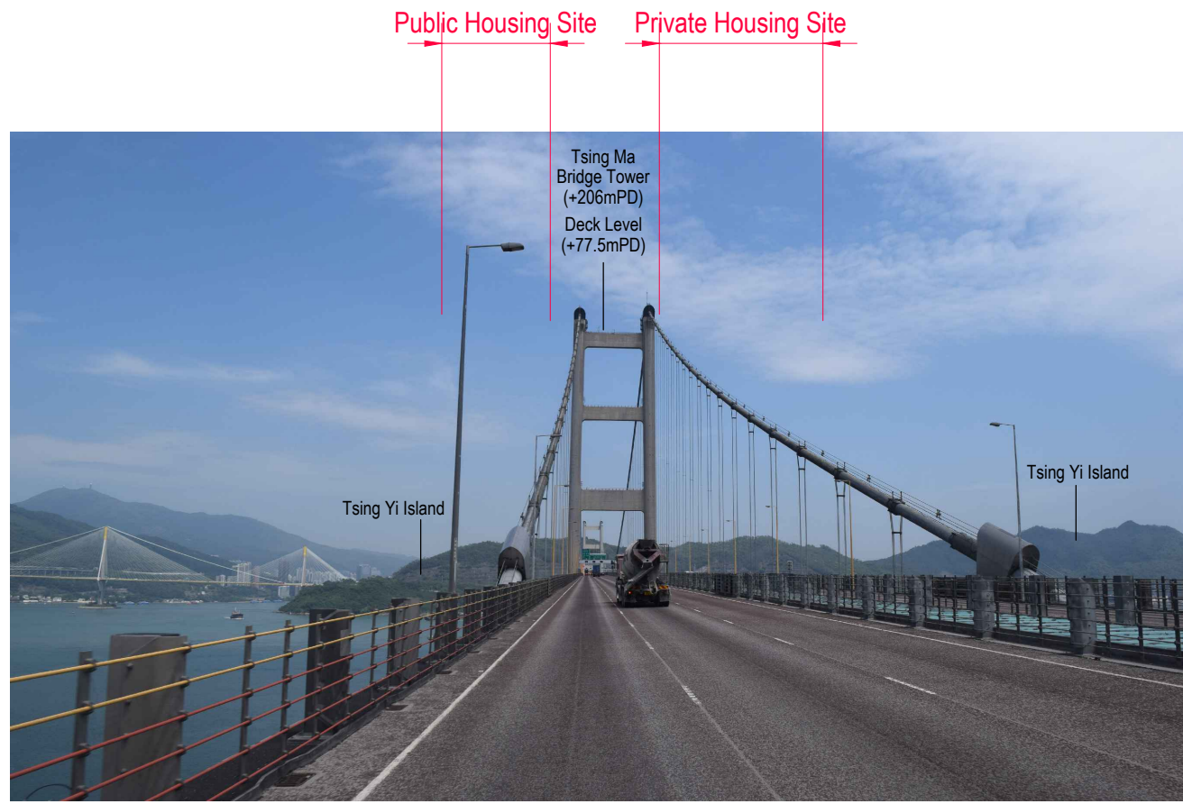
VP5 Original View from Tsing Ma Bridge Deck (Eastbound)
